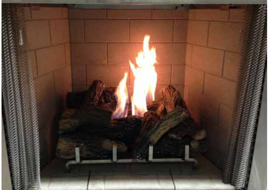
Figure 23 - Proper Burner Flame Appearance
