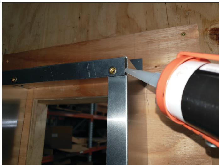
Figure 2.6, Appliquez le scellant silicone aux coins
