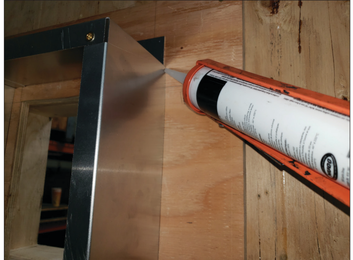
Figure 2.7, Silicone Perimeter
