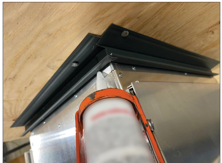
Figure 2.9, Silicone Finishing Materials
