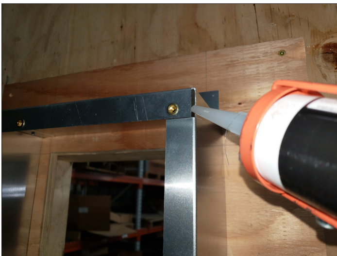
Figure 2.6, Appliquez le scellant silicone aux coins
