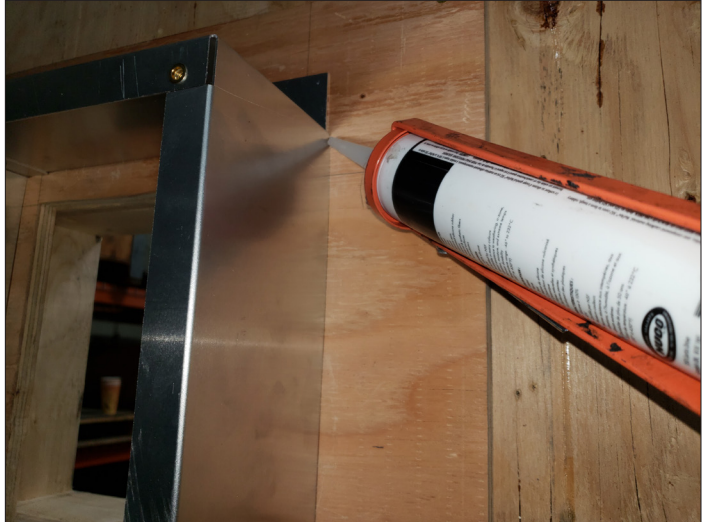
Figure 2.7, Silicone Perimeter
