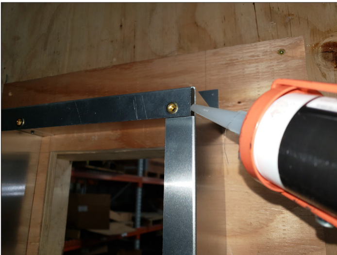
Figure 2.6, Silicone Corners
