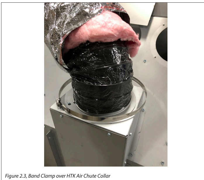
Figure 2.3, Band Clamp over HTK Air Chute Collar
