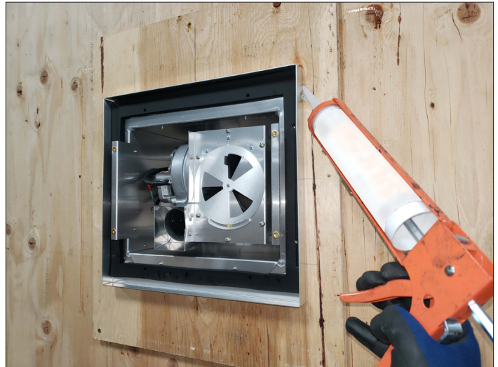
Figure 3.20, Silicone around the Cap Base
