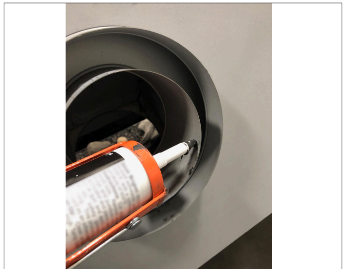
Figure 2.2, Apply Sealant to Inner Exhaust on Fireplace
