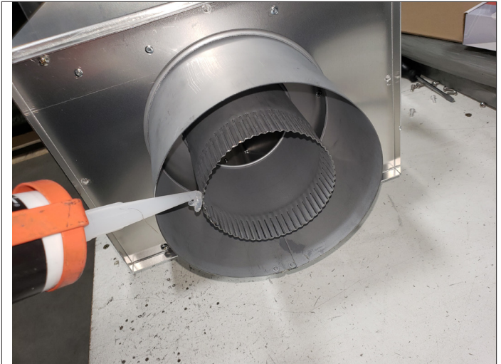
Figure 2.1, Silicone Inner Exhaust on Power Vent Assembly
