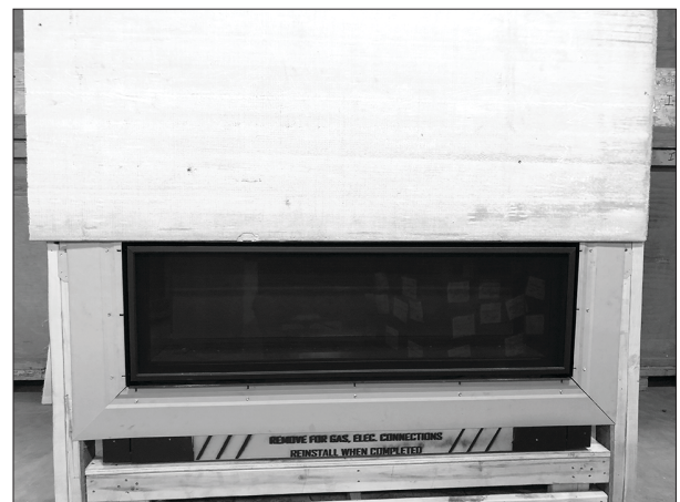
Figure 4.9, Installed Panels and Non-Combustible Material
