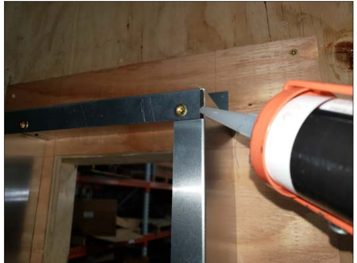
Figure 2.9, Appliquez le scellant silicone aux coins
