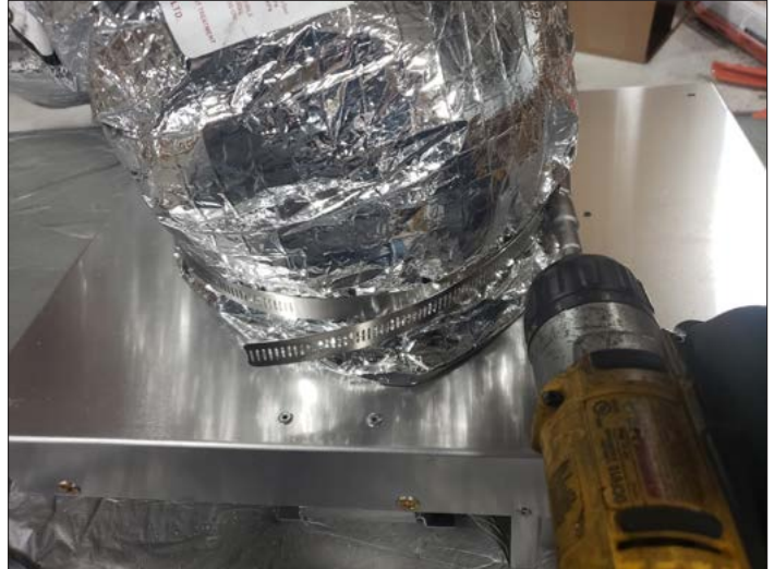
Figure 2.17, Liner Installed with Band Clamp
