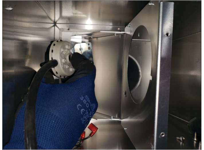
Figure 5.9, Vacuum Switch Removal
