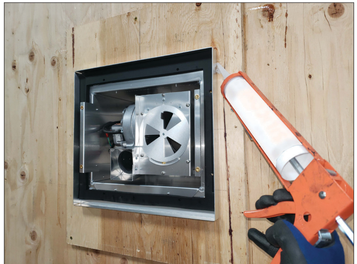
Figure 3.20, Silicone around the Cap Base
