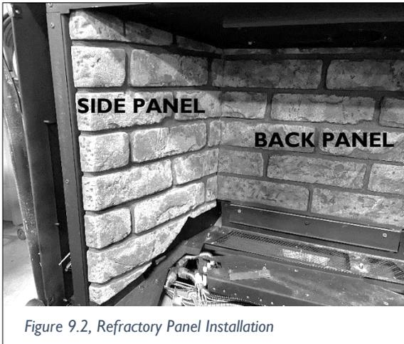
Figure 9.2, Refractory Panel Installation
