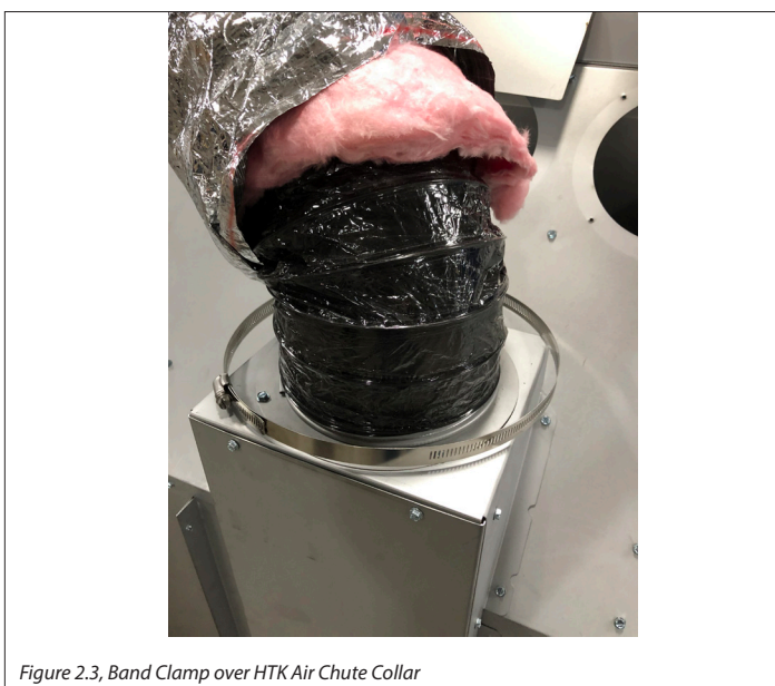
Figure 2.3, Band Clamp over HTK Air Chute Collar
