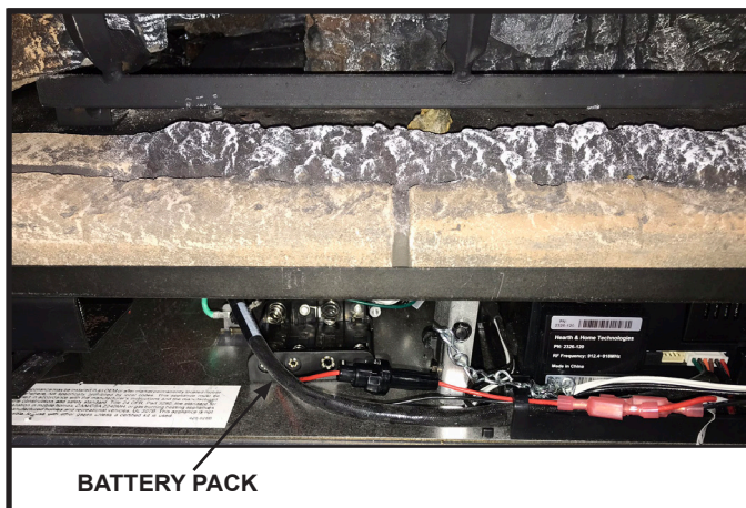
Figure 6.3 Battery Pack Installed
