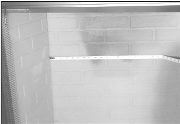
Figure 2.1 Measure Firebox
