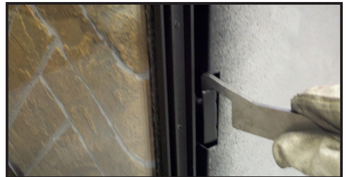
Figure 11.7. Securing Side Glass Clips
