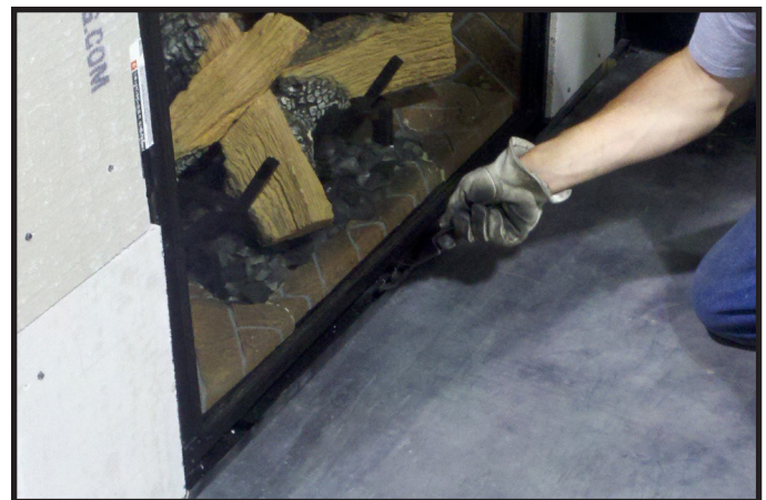
Figure 11.8. Securing Bottom Glass Clips
