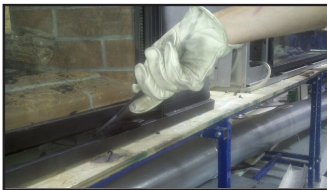
Figure 11.3. Inserting Glass Clip Tool
