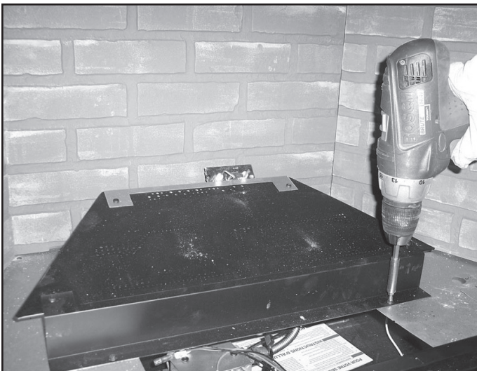
Figure 14.28 Remove Screws Attaching Front Burner Support
