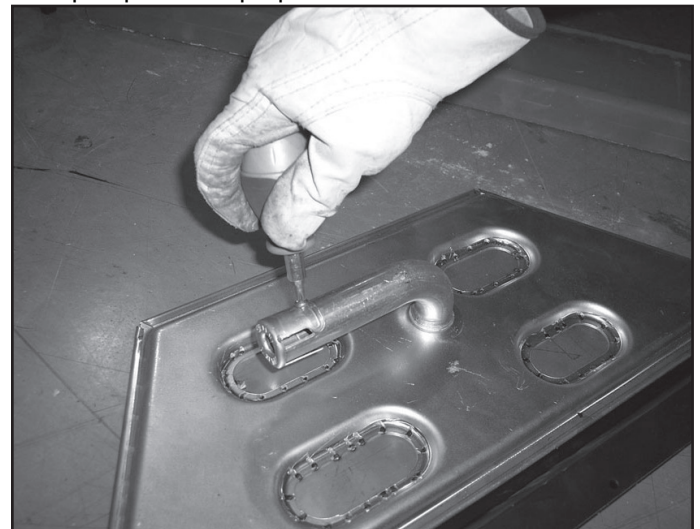
Figure 14.31 Adjust Air Shutter
