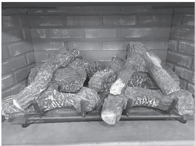
Figure 14.20 Final Log Placement
