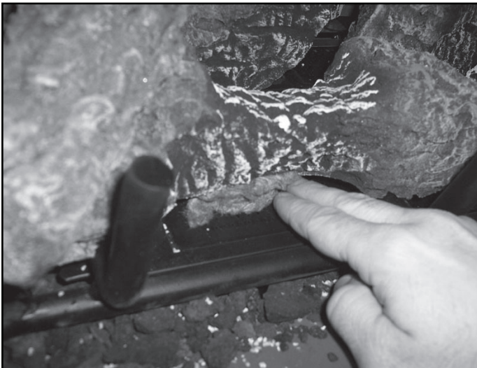
Figure 14.24 Placement of Rockwool Under Front Logs
