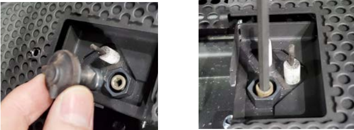
Figure 13.e Removing the pilot hood, orifice
