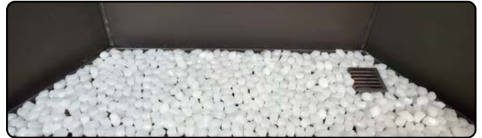
Figure 24.bb Completed firestone installation
