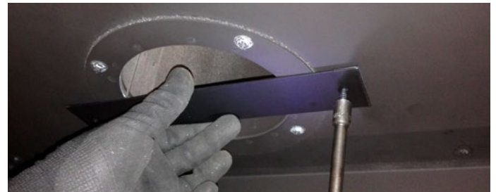
Figure 8.b.c Restrictor plate Installation
