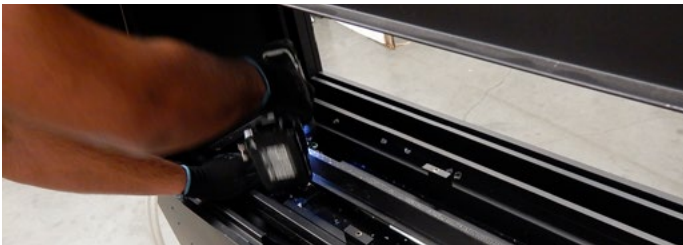
Figure 12.d Removing the Burner screws
