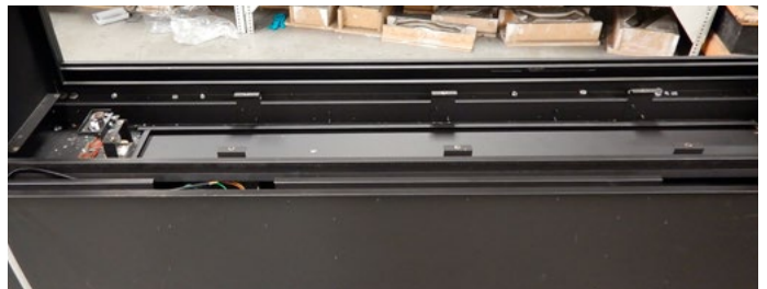
Figure 12.e Removing the Burner
