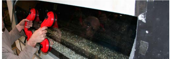
Figure 11.c Window Removal (using glass lifting tools).
