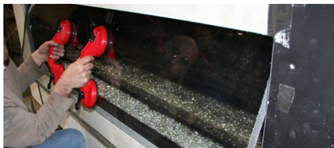
Figure 11.c Window Removal (using glass lifting tools).
