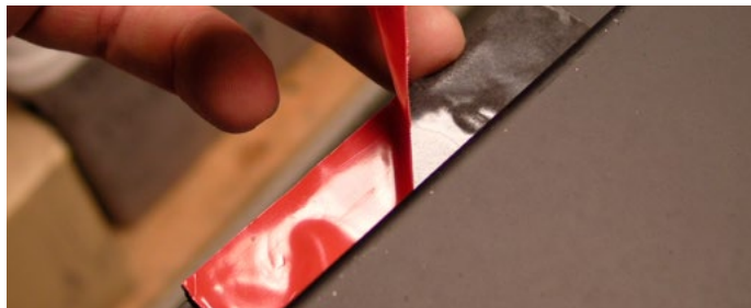
Figure 5.12b Peeling self-adhesive tape
