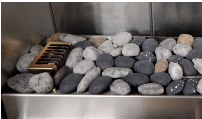
Figure 70 Ensure the stones DO NOT cover the pilot.
