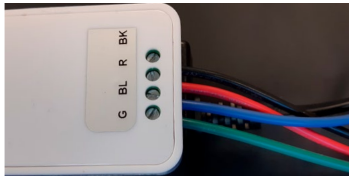
Figure 48 Wiring the LED receiver
