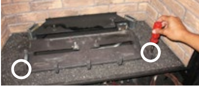
Diagram 1: Remove the left and right screws.
