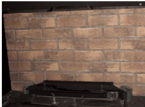
Back Panel Installed
