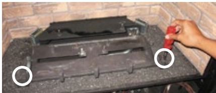
Diagram 1: Remove the left and right screws.
