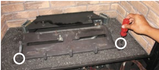
Diagram 1: Remove the left and right screws.
