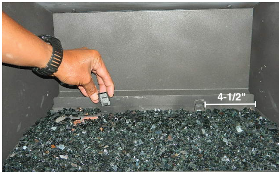
Log bracket install
