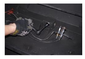
9) Remove pilot retainer clip with pliers and pull off the pilot cap to expose the pilot orifice.
