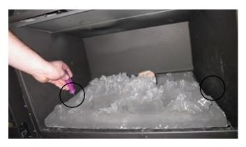
3) Lift the Burner slightly while pulling forward to clear the mixing tube.
