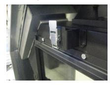
Lift the screen up so that the bottom of the screen clears the bottom of the fireplace opening.
