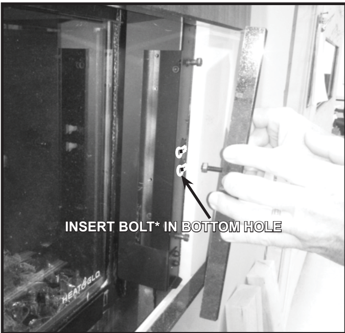
Figure 10.25. Install Side Granite Pieces
