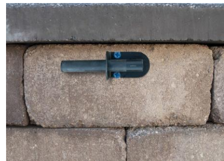
Figure 6.5 – Fasten down the bracket
