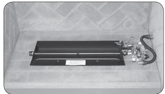
Fig. 16-2 Center burner in firebox
