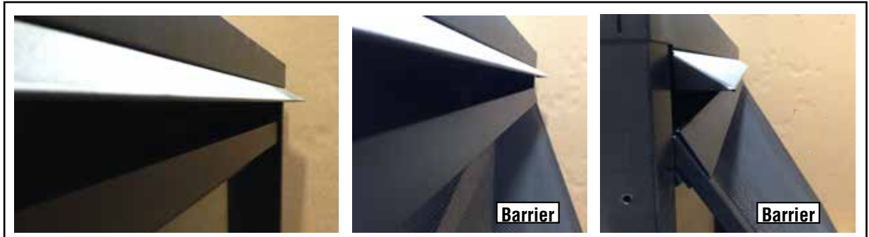
Figure 47A - Slide Barrier into Upper Trim Panel
