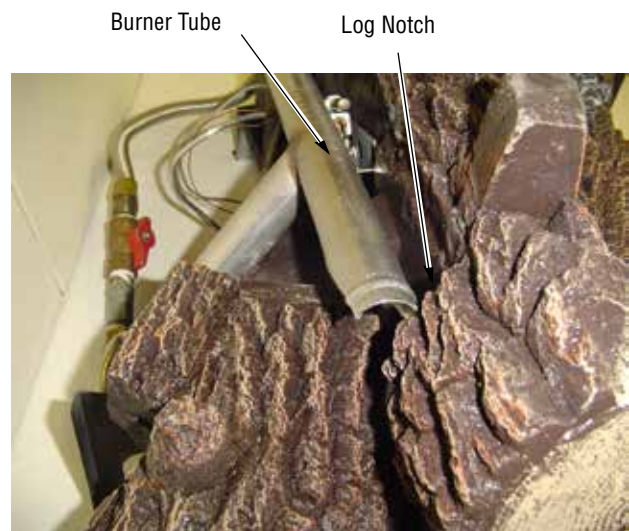
Figure 22A - Installing Middle Split Log Rear Top Side View
