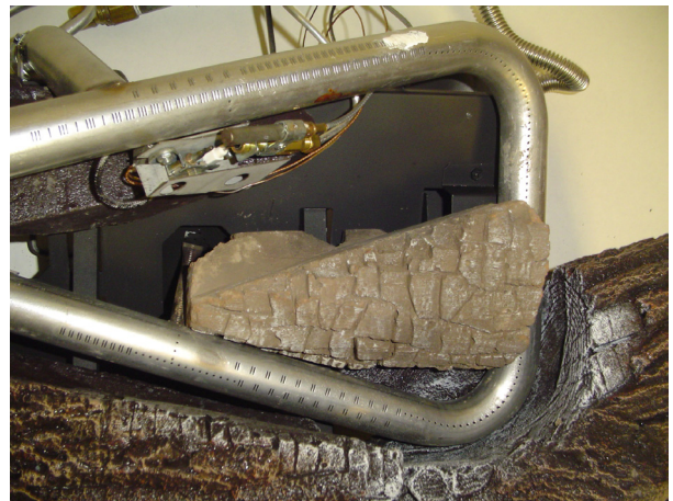
Figure 21A - Installing Charred Log Top View
