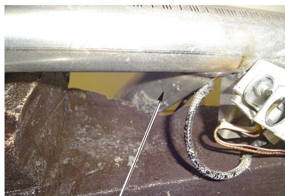
Figure 19B - Installing Back Left Log (D-018) Rear View
