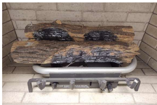
Figure R - Install Middle Log
