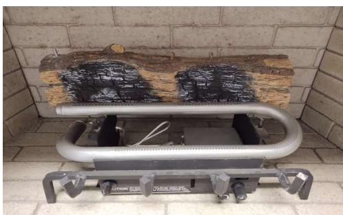
Figure P - Install Rear Log
