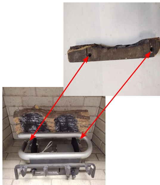
Figure Q - Middle Log Placement
