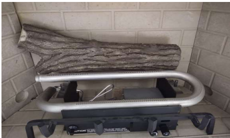
Figure B - Install Rear Log
