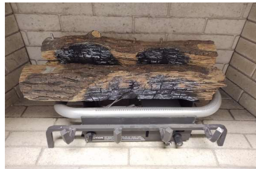
Figure R - Install Middle Log
