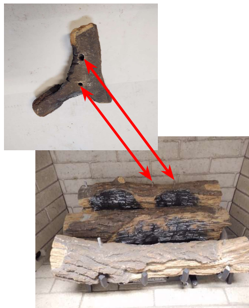
Figure U - Middle Log Placement
