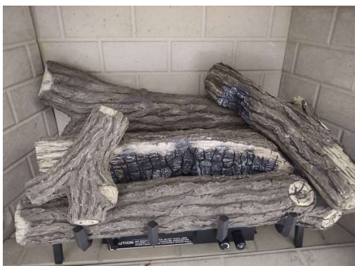
Figure K - Install Top Left Log
