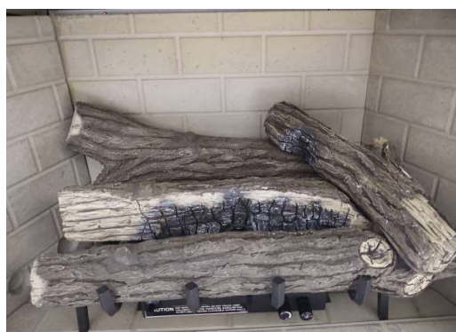
Figure H - Install Right Top Log
